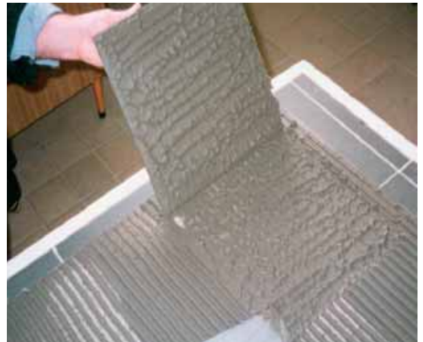
Fig. 5 - Buttering- Floating glueing method
